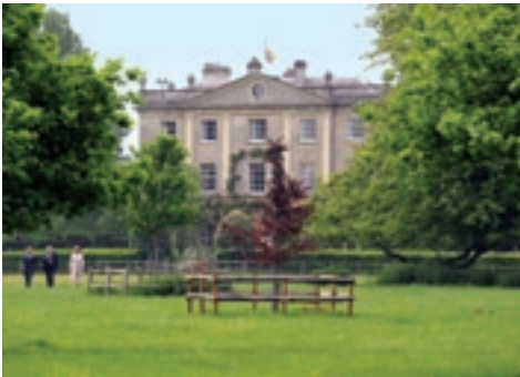
ABOVE FROM TOP TO BOTTOM Clarence House, where more efficient boilers have been installed.
