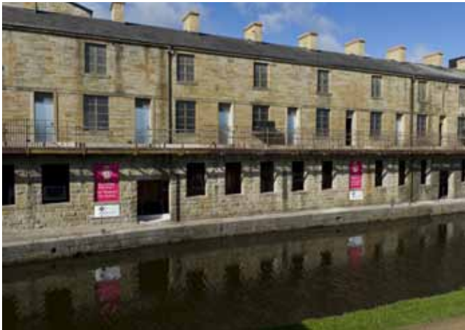
Renovation of The Weavers' Triangle – Slater's Terrace in Burnley
